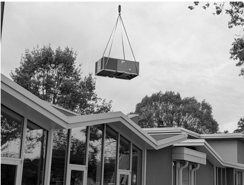
One of the new HVAC compressors is lifted into place on the roof of the education building.
